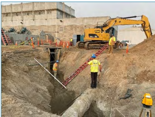
Pipe bedding placement at 12-inch grit drain trench
