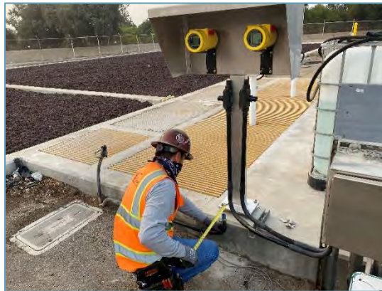
Blower duct flowmeter conduit installation
