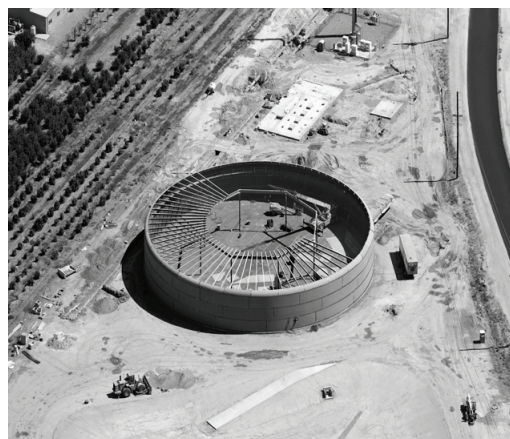
Aerial view of the West Tank under construction
