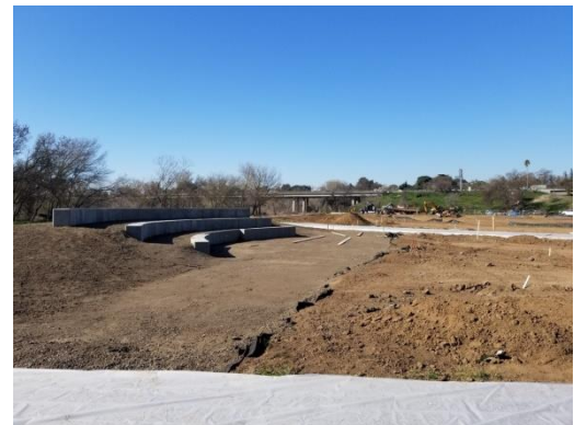
Outdoor Classroom with Pervious Concrete Trails Completed
