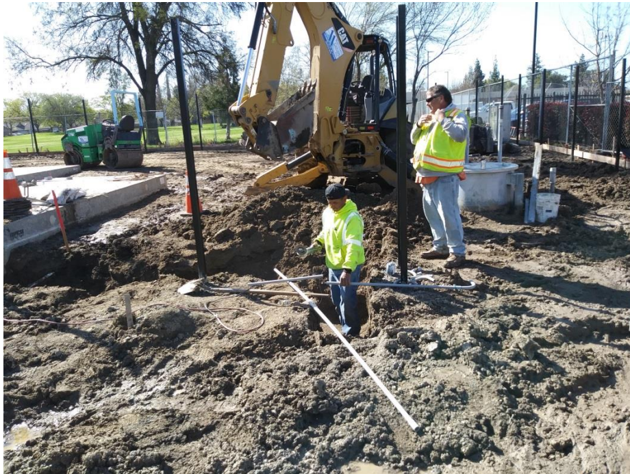
Hahn and Rumble Lift Station Improvements
