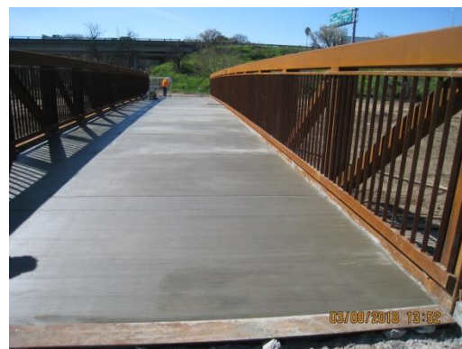
Pedestrian/Light Vehicle Bridge with Concrete Deck Poured
