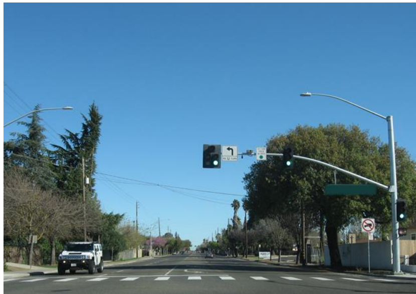
Upgraded Traffic Signal
