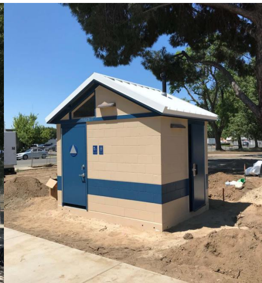
New Restroom at Pike Park
