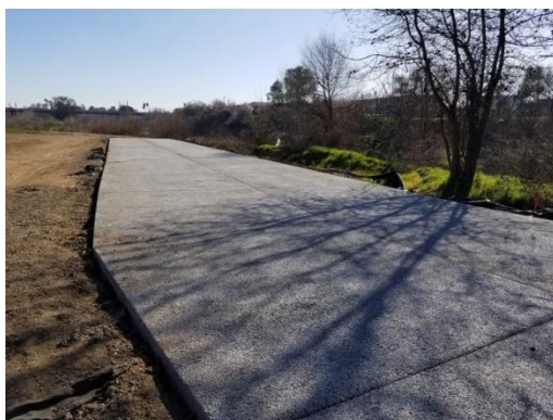
Observation Deck with Completed Pervious Concrete
