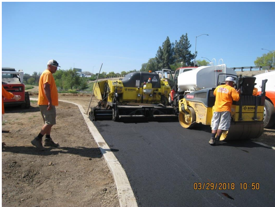
Cannery Segregation Line Diversion Structure
