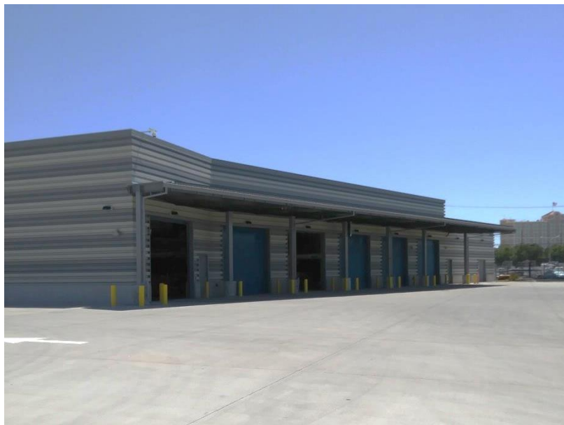
Bus Maintenance Facility Canopy
