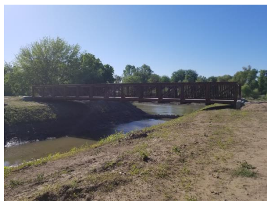
Pedestrian/Light Vehicle Bridge
