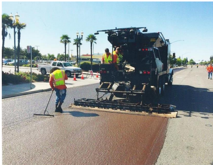
Slurry Seal Project
