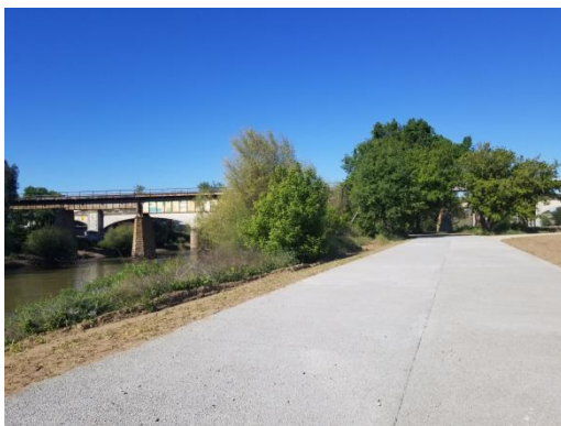
Observation Deck with Completed Pervious Concrete
