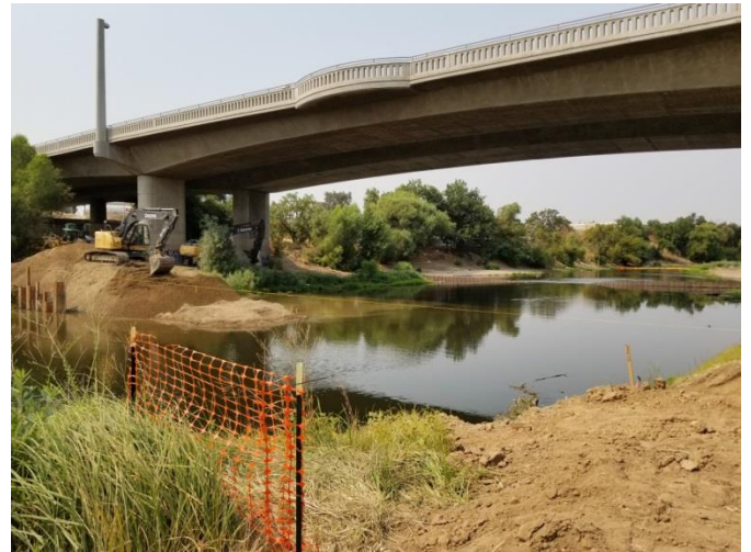
Temporary Cofferdam Installation
