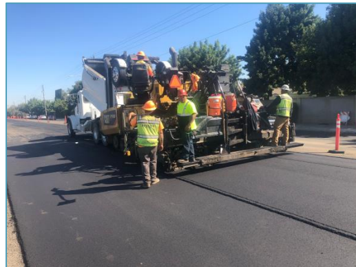
Leveling Course Work
