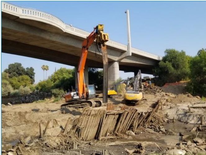
Removal of twenty foot long sheet piles from Remnant Dennett Dam
