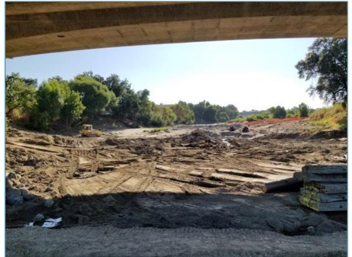
Removal of Old 9 th Street Bridge footings from Tuolumne river bed
