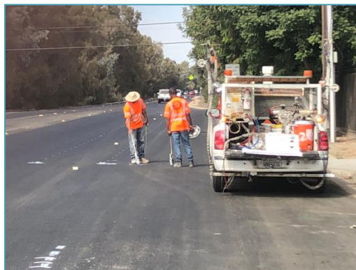
Contractor Cat Tracking Traffic Lane Line Locations
