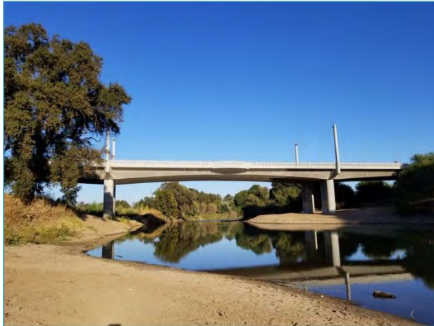
View of Dennett Dam Removed
