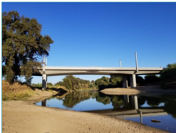
View of Dennett Dam Removed
