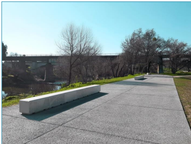
New benches and landscaping recently seeded with native plant species.
