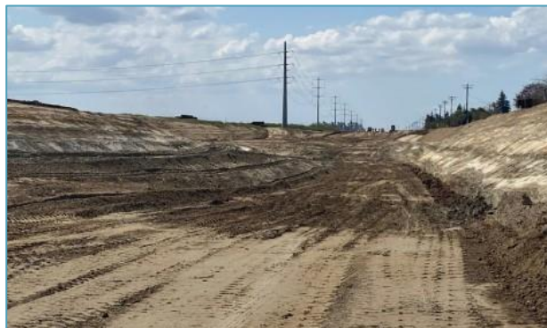
Rosemore Avenue Excavation
