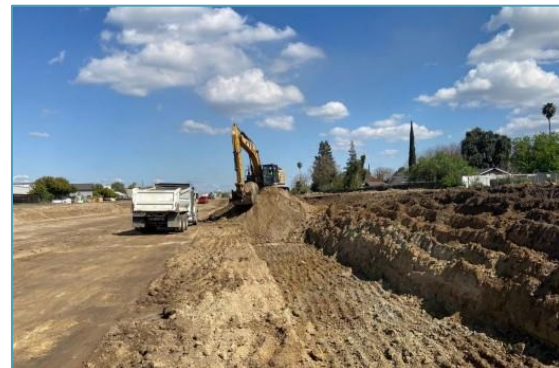
Roadway Excavation East of Carpenter
