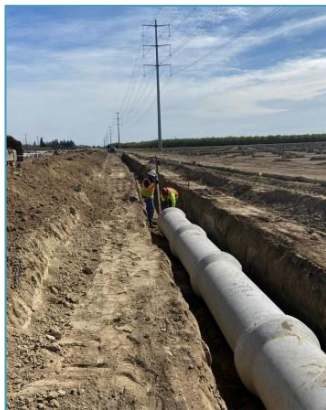
Drainage System 10 Installation
