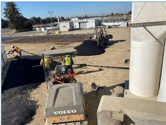
AC paving operations on south side
