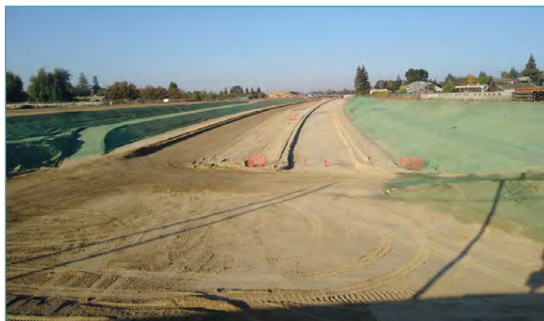
Carpenter Bypass Alignment
