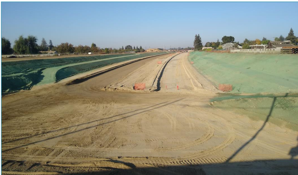
Carpenter Bypass Alignment
