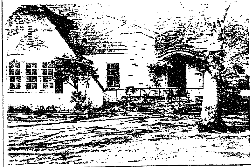
P5a. Photograph or Drawing (Photograph required for buildings, structures, and objects.)
