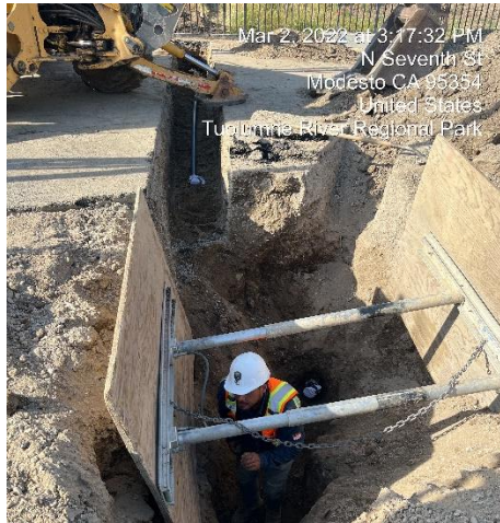
Placement of electrical conduits for diversion structure biofilter
