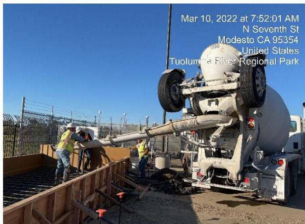
Concrete placement for diversion structure biofilter equipment pad
