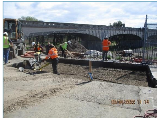
Subgrade prep for Biofilter equipment pad
