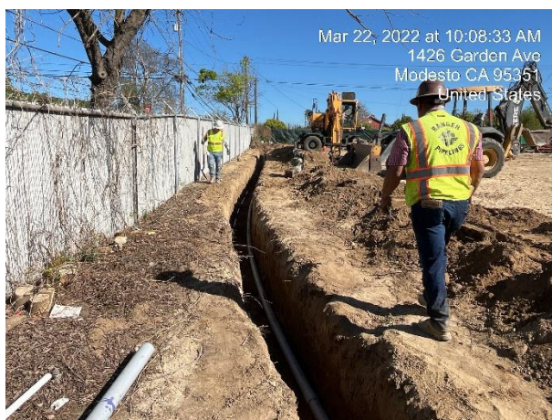
Temporary utilities installation for construction trailers
