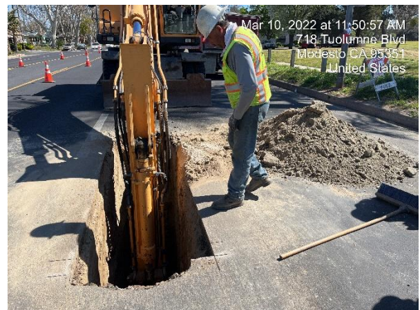
Potholing to expose existing utilities on Tuolumne Boulevard
