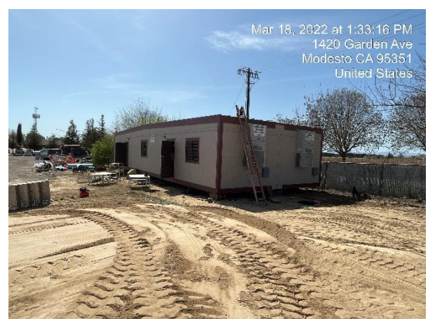
Construction trailer at Sutter Plant staging area
