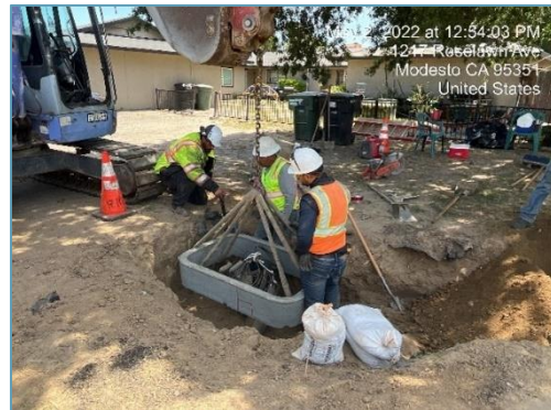
Placement of AT&T pull box components at Colorado Avenue and Garden Avenue
