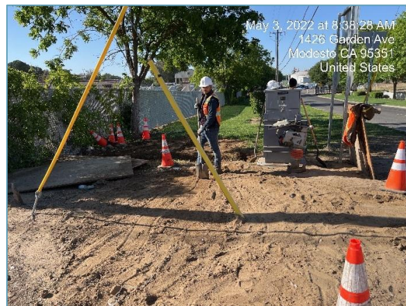
Backfill of temp utility trenches at job trailer area
