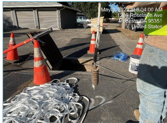
Mandrel testing of rerouted MID electrical conduit (passed)
