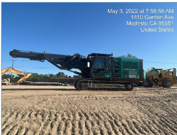
Pile driver for shoring system
