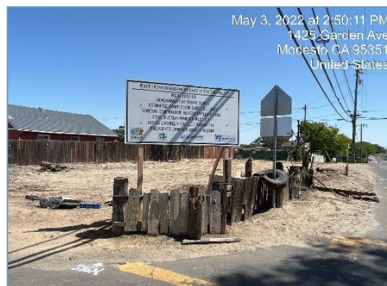
Sign at Garden Avenue and Sutter Avenue facing west
