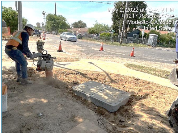
Backfilling AT&T junction box at Colorado Avenue and Garden Avenue
