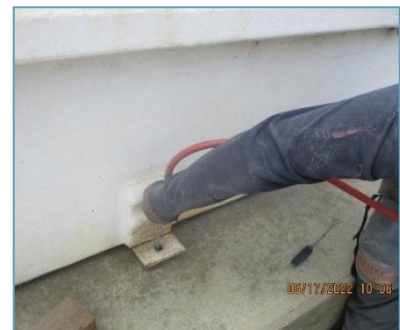
Compressed air (>90 psi) cleanout of anchor bolt holes at biofilter
