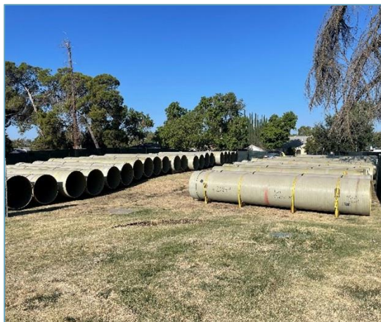
Staging of couplings at Muni Golf Course
