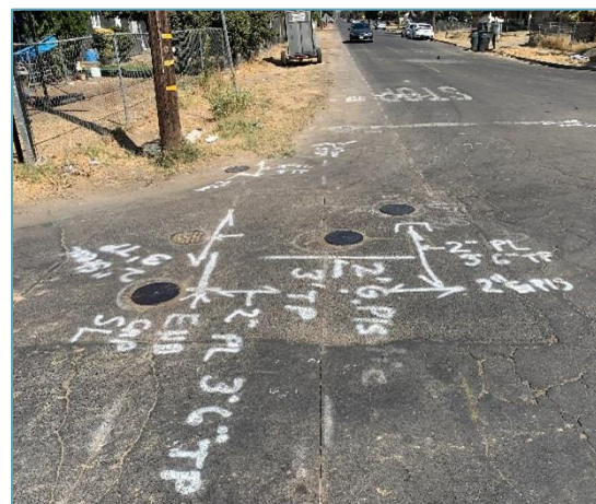
Markings of existing utilities at the intersection of Colorado Avenue and Garden Avenue
