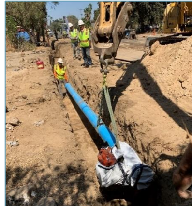
Installation of 8-inch water main line on Colorado Avenue
