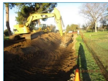
Backfill of 18-inch pipeline
