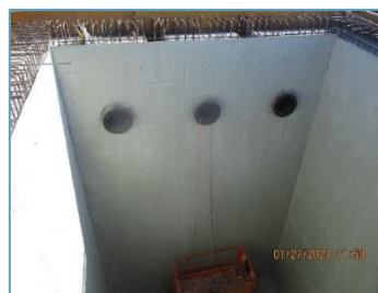
Stripping of wet well interior wall panels
