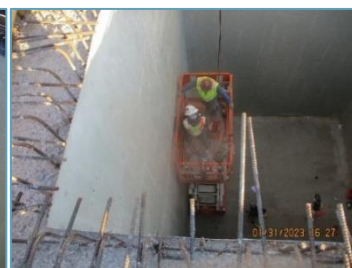
Repair of HDPE liner
