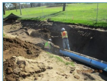
Removal of pipeline section that floated during storms
