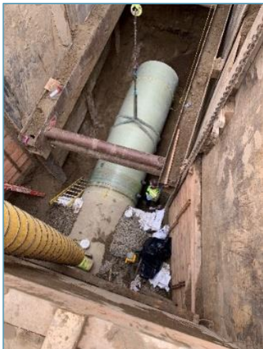
Installation of first segment of 60-in. FRPMP
