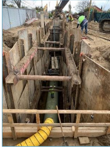
Preparation for slurry encasement
