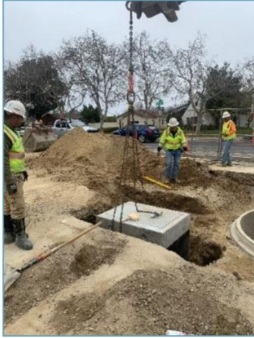
Installation of fiber optic pull box on Tuolumne Boulevard
