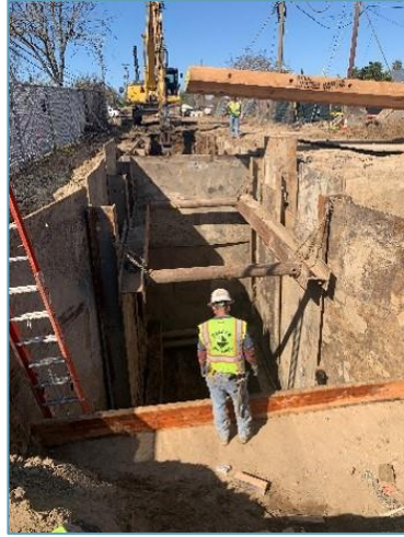
Shoring placement at Sutter Avenue vacant lot
