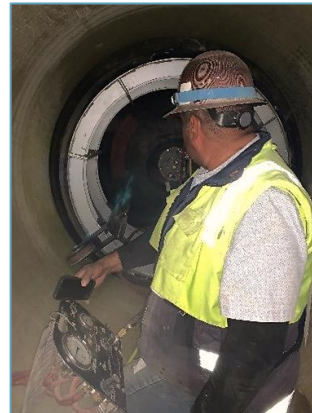
FRPMP joint air pressure testing operations
