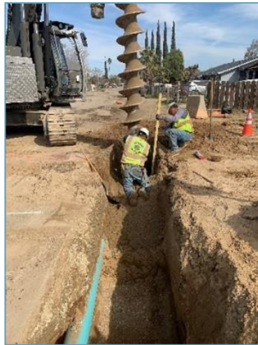
Auguring on Garden Avenue
