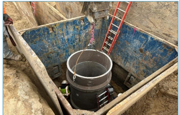
8-inch Sewer Manhole Installation
