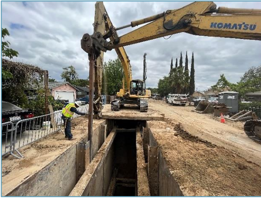
Placement of shoring on Garden Avenue
