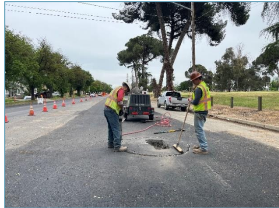
Raising manhole grade rings along Tuolumne Boulevard
