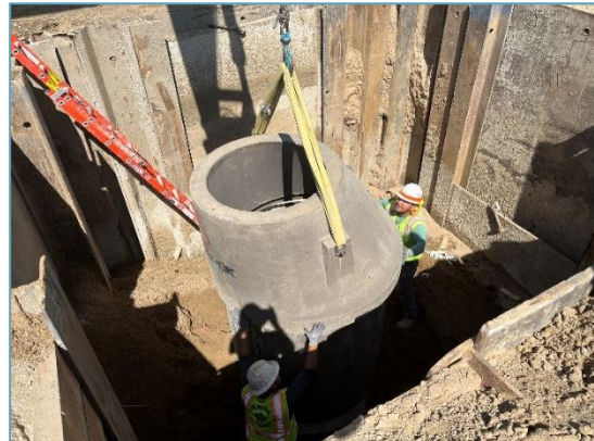
Raising manhole grade rings along Tuolumne Boulevard
