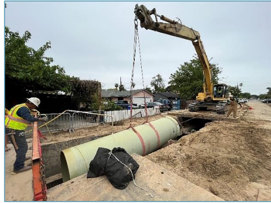
60-inch FRPMP placement along Garden Avenue
