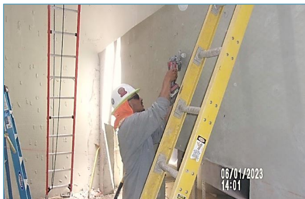
Repair of baffle wall HDPE liner
