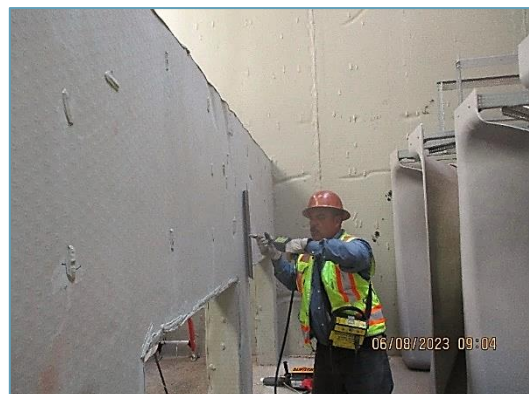
Testing of HDPE liner
