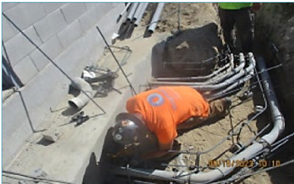
Rebar placement for duct bank
