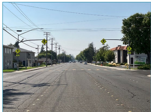
Upgrade lighted crosswalks
