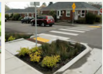
Curb bulb-outs and ADA ramps
