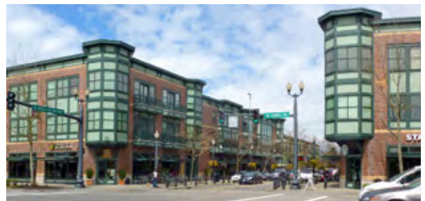
Figure 2.11 Orenco Station, Oregon is a reputed example of a walkable, mixed-use town center at a light rail station.
