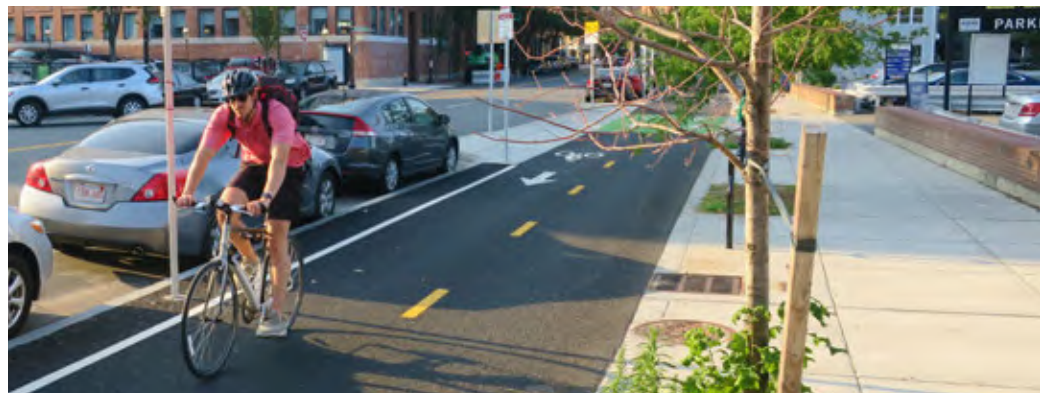
Figure 3.15 A two-way protected bikeway as an example of the recommended improvements for 9th Street
