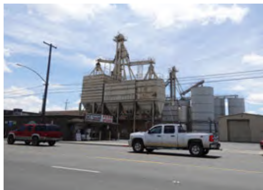
Figure 1.20 Lot dimensions range from small and regular (far left) to large and irregular (left), and these characteristics help to inform redevelopment strategies.
