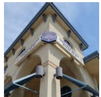
Figure 5.4 Existing civic uses in downtown add to its character and signify regional importance.
