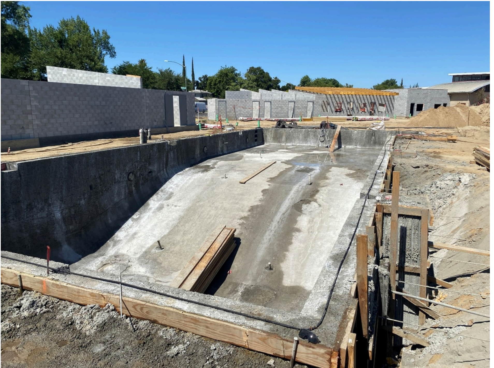
CHAVEZ PARK POOL INSTALLATION
