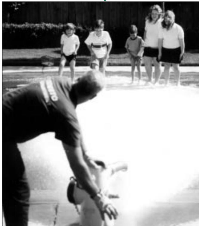
It was a pre-summer splash for some of Modesto's youth as Modesto Fire Department crews conducted routine servicing of city fire hydrants. The hydrant stems are opened to examine water pressure and valves are checked for leaks. The routine inspections help fire department personnel identify potential problems so that fire suppression efforts are not interrupted during emergencies.
