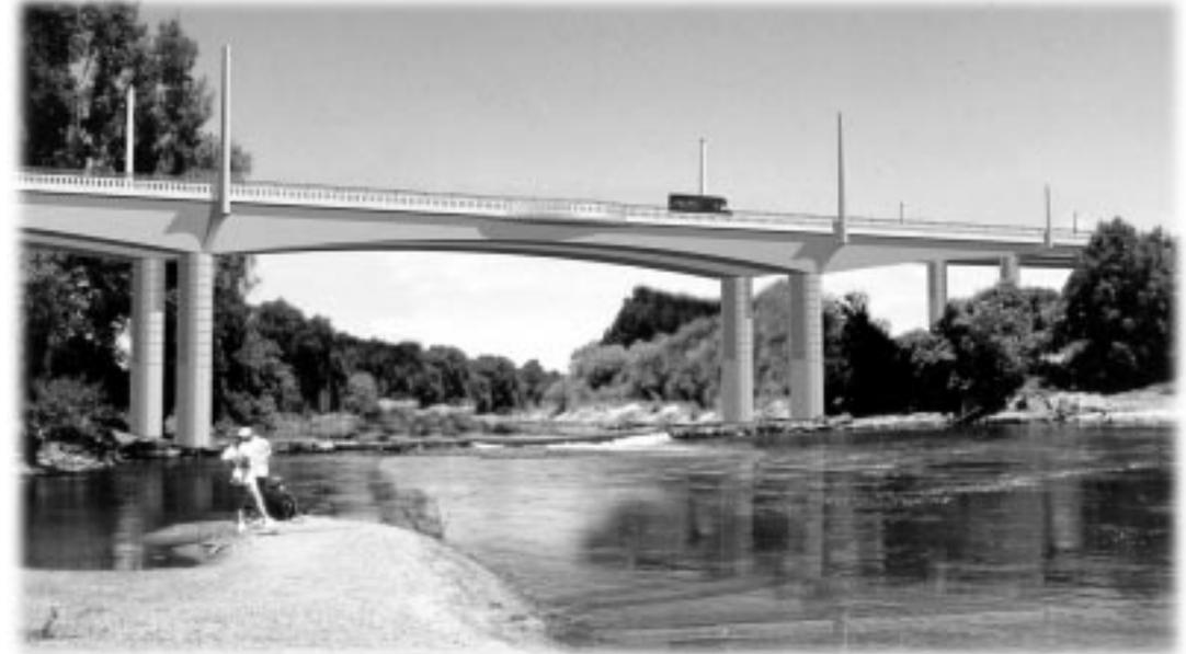
*Architectural renderings depict a concrete box girder bridge that is supported by columns on large diameter piles.*
