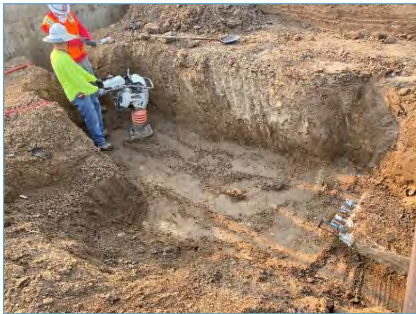
Dryden Box duct bank trench subgrade prep
