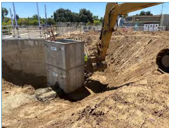
Slurry placement at 20-inch return line subgrade vault connections
