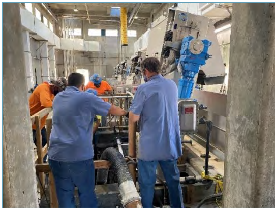
Clean out of channel 5 for installation of barscreen
