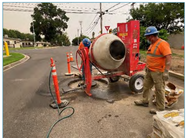
Concrete collar placement at Sutter Trunk near plant entry
