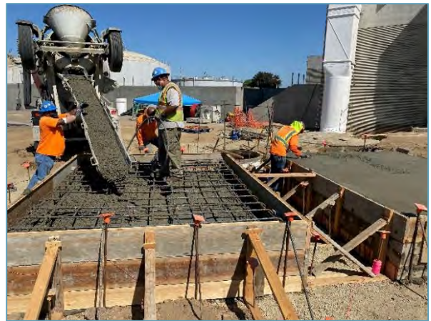
Concrete placement at equipment pads south building
