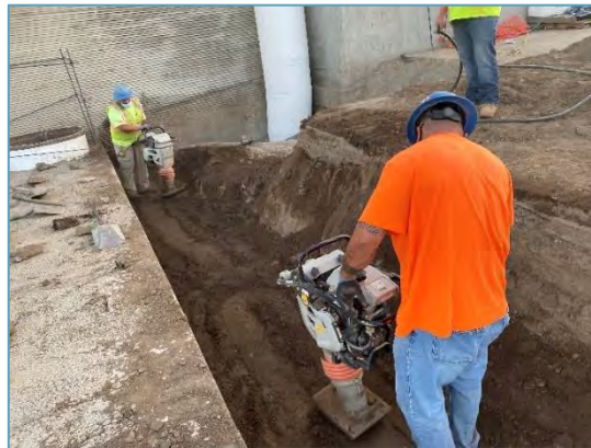
Backfill/compaction operations
