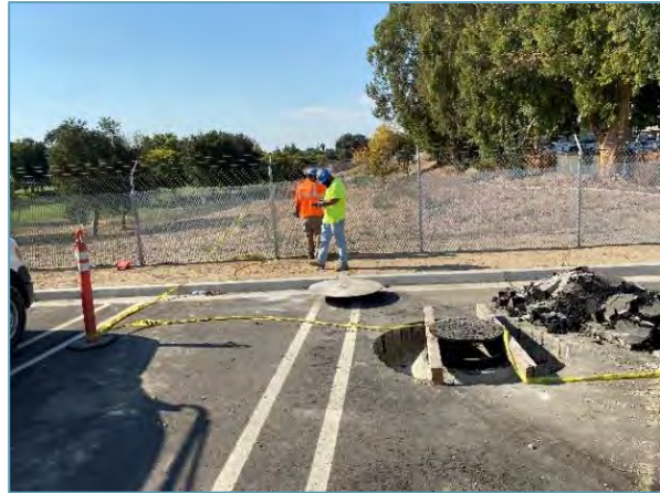
Prep for concrete collar placement
