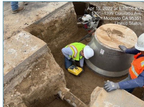
Compaction testing at Colorado Avenue and Garden Avenue
