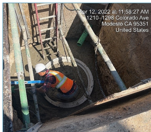
Concrete placement at foundation
