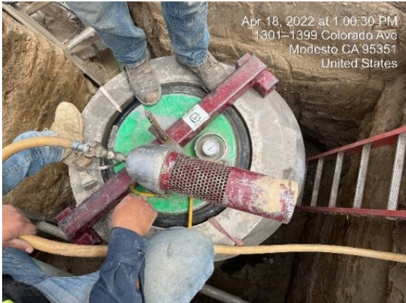
Vacuum testing at Colorado Avenue and Garden Avenue
