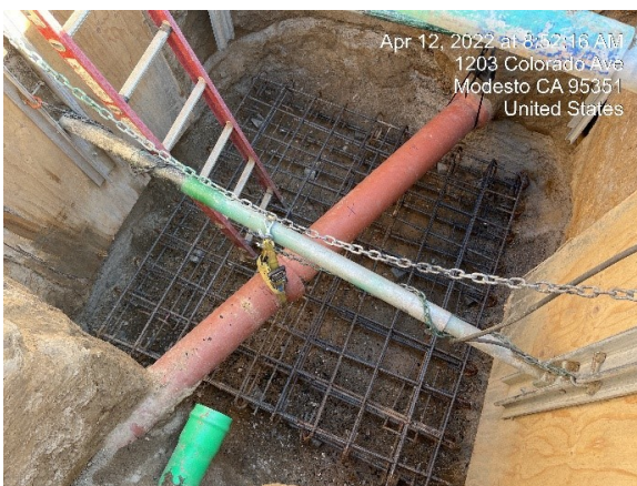
Foundation rebar
