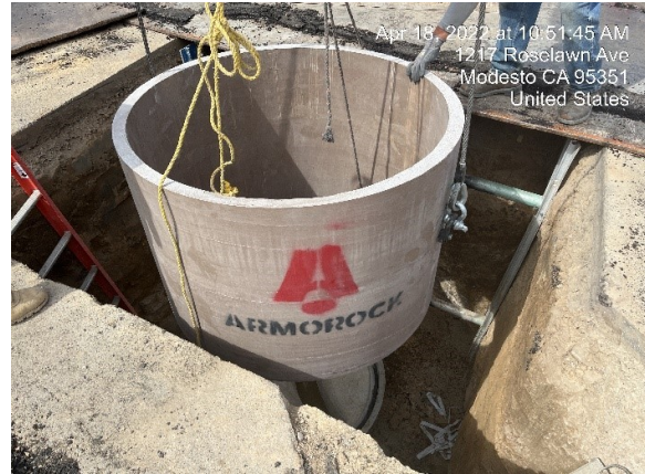
Installation of Armorock at Colorado Avenue and Garden Avenue
