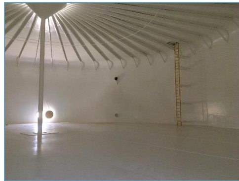
Tank 5 Interior Complete
