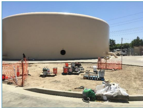
Tank 5 Exterior Coating
