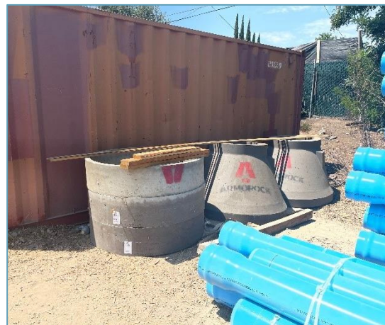
Armorock MH materials for installation at junction structures
