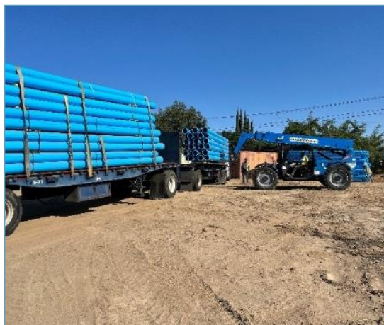
Delivery of PVC C900 waterline pipe
