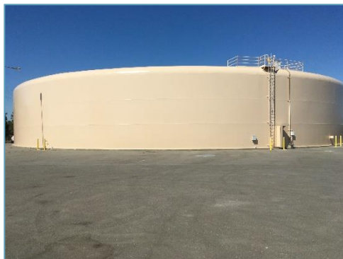
Tank 12 Exterior Final Coating
