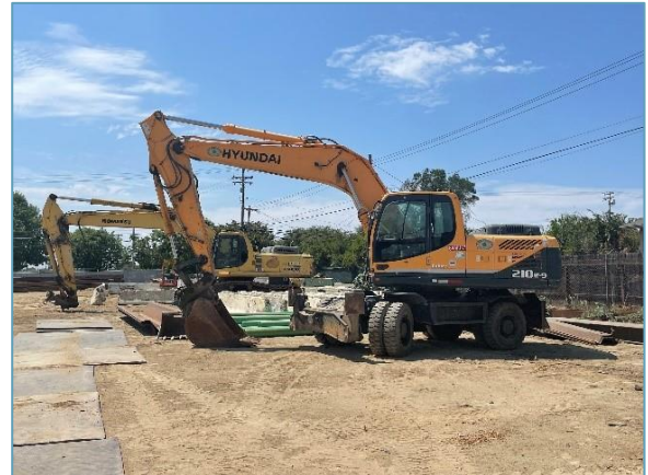
Equipment mobilized in preparation for pipe installation
