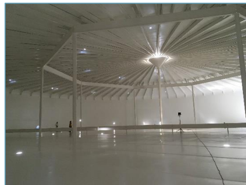
Tank 12 Interior Complete
