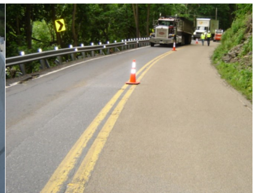
High Friction Surface Treatment applied to Pennsylvania Department of Transportation Route 611
