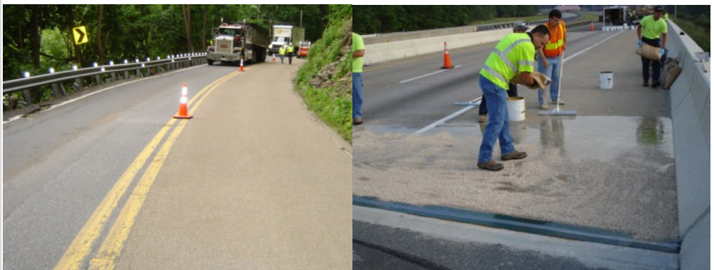
High Friction Surface Treatment applied to Pennsylvania Department of Transportation Route 611
