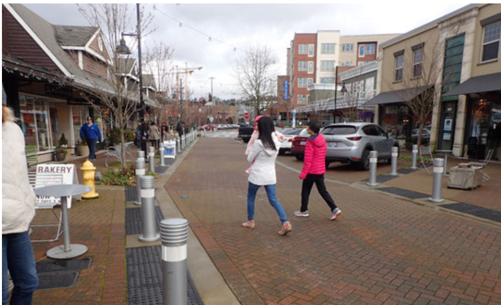
Figure 4.10 Pedestrian-priority streets An example of a curbless or “flush” street in Redmond, WA with delineated spaces for different modes, pedestrian-scale lighting, and outdoor activated business or dining areas.
