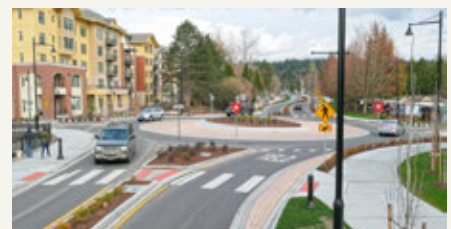
Figure 4.16 Example of a roundabout
