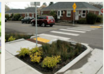
Curb bulb-outs and ADA ramps
