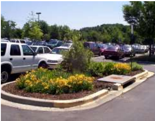
Figure III-14: Photograph of Parking Lot Inlet
