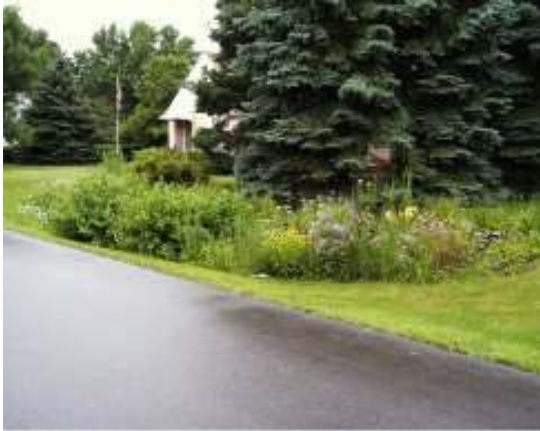
Figure III-13: Photograph of Biological swale
